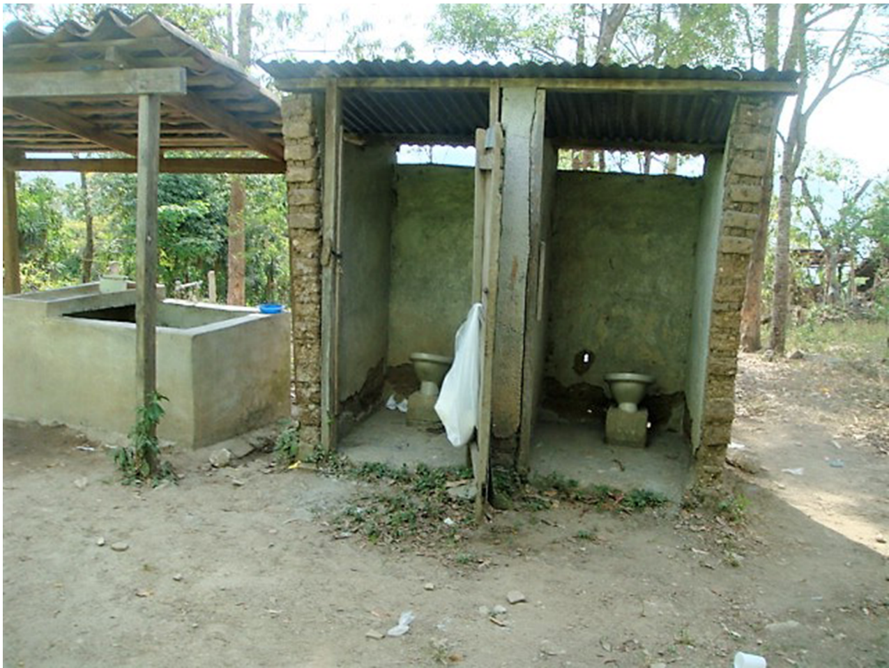
Figure 2 An open and uncovered water source within meters of the village latrine or outhouse facility.
